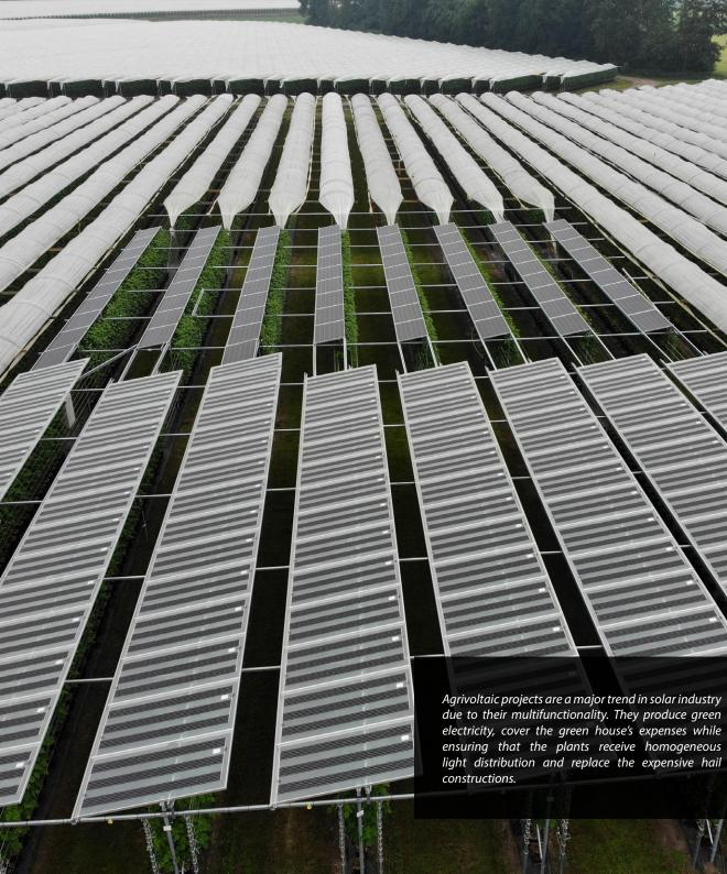
Bifacial Monocrystalline PV Modules with Transparent Backsheet
